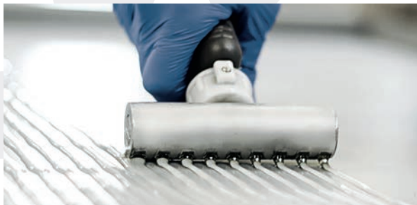
Applying the adhesive
